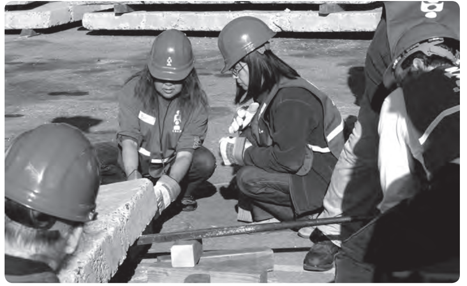
SNAP participants learn how to lift and move heavy debris like this concrete slab
