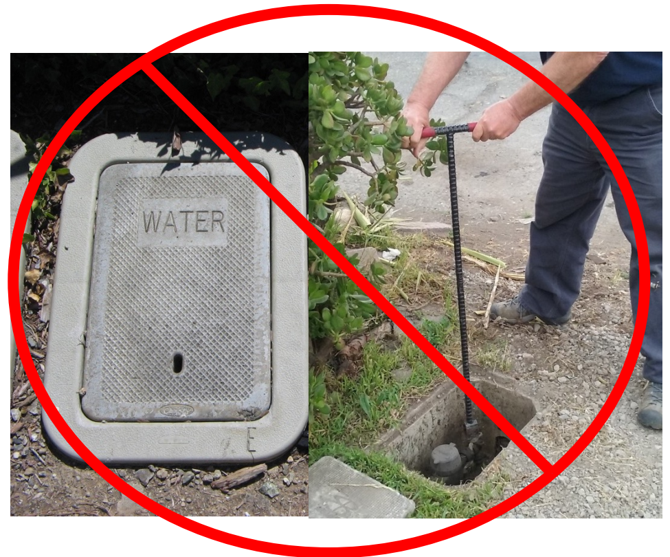
Not the street (water meter)
